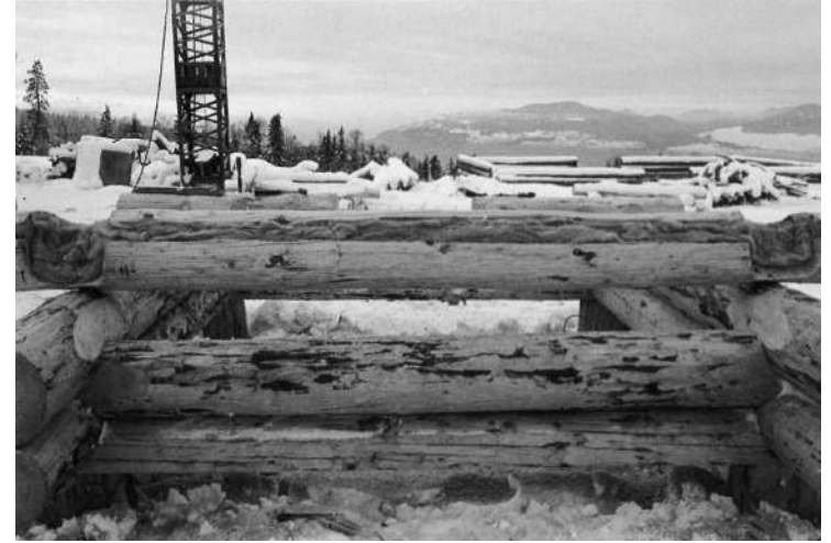
STEP 28: The entire log, from notch-to-notch, is insulated.
