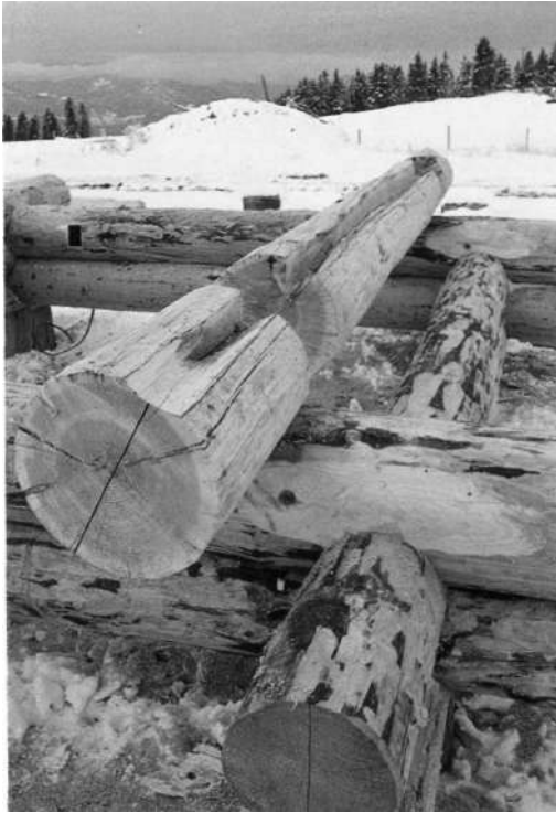
STEP 26: The LATERAL GROOVE is completed and final touch-up may be done with either an axe, chisel or slick.
