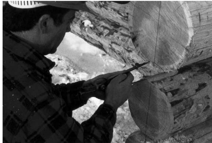
STEP 10: Scribe the end cove, always keeping the dual level bubbles PERFECTLY LEVEL.
