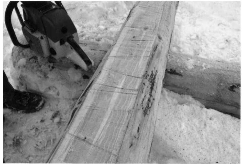
STEP 16: Because of a pivoting motion, small 'ridges' will occur along the cut surface of the log.
