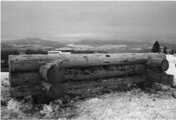
STEP 29: The log is rolled back and re-aligned, using the 'Plumb Line' as the reference mark.
