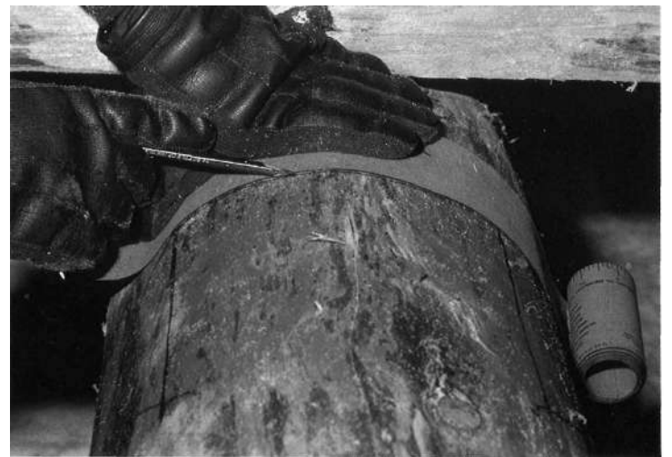
STEP 10: A flexible guide is a useful straight-edge for drawing the line.
