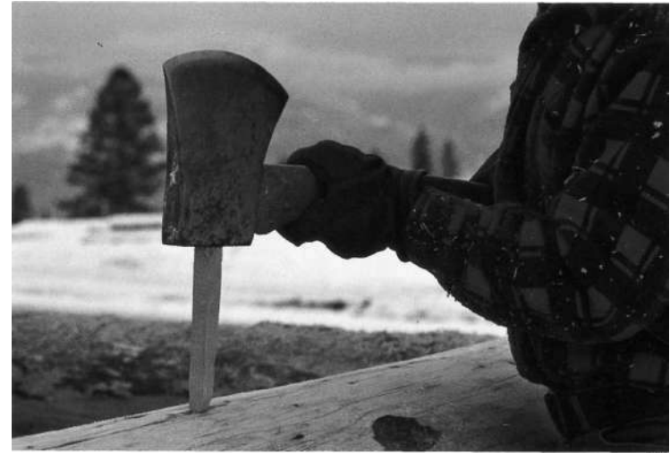
STEP 30: Hardwood wedges are driven into the upper surfaces of the log approximately every 24 inches (62 cm). This is to pre-stress the log and localize the checking to the top surface of the log.
