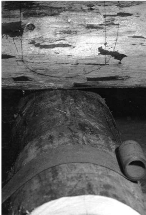
STEP 9: The final layout is done by connecting all opposing "critical points" with a pencil line.
