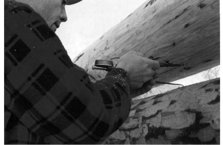
STEP 9: Scribe the lateral groove, always keeping the dual level bubbles PERFECTLY LEVEL.
