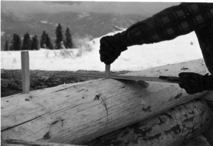
STEP 31: The wedges are trimmed.
