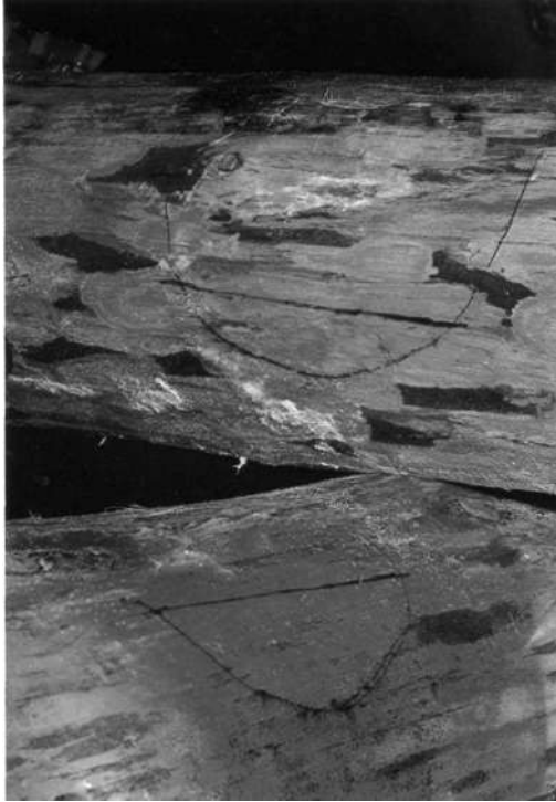
STEP 8: The joist is rolled back.
